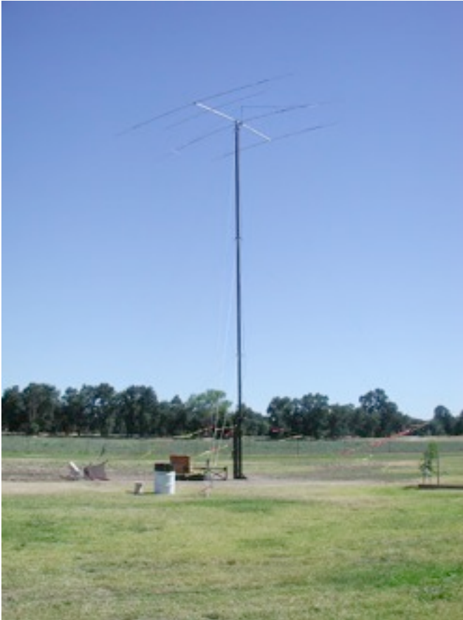
Cushcraft antenna on tower Photo by Greg Lane KA6BID
